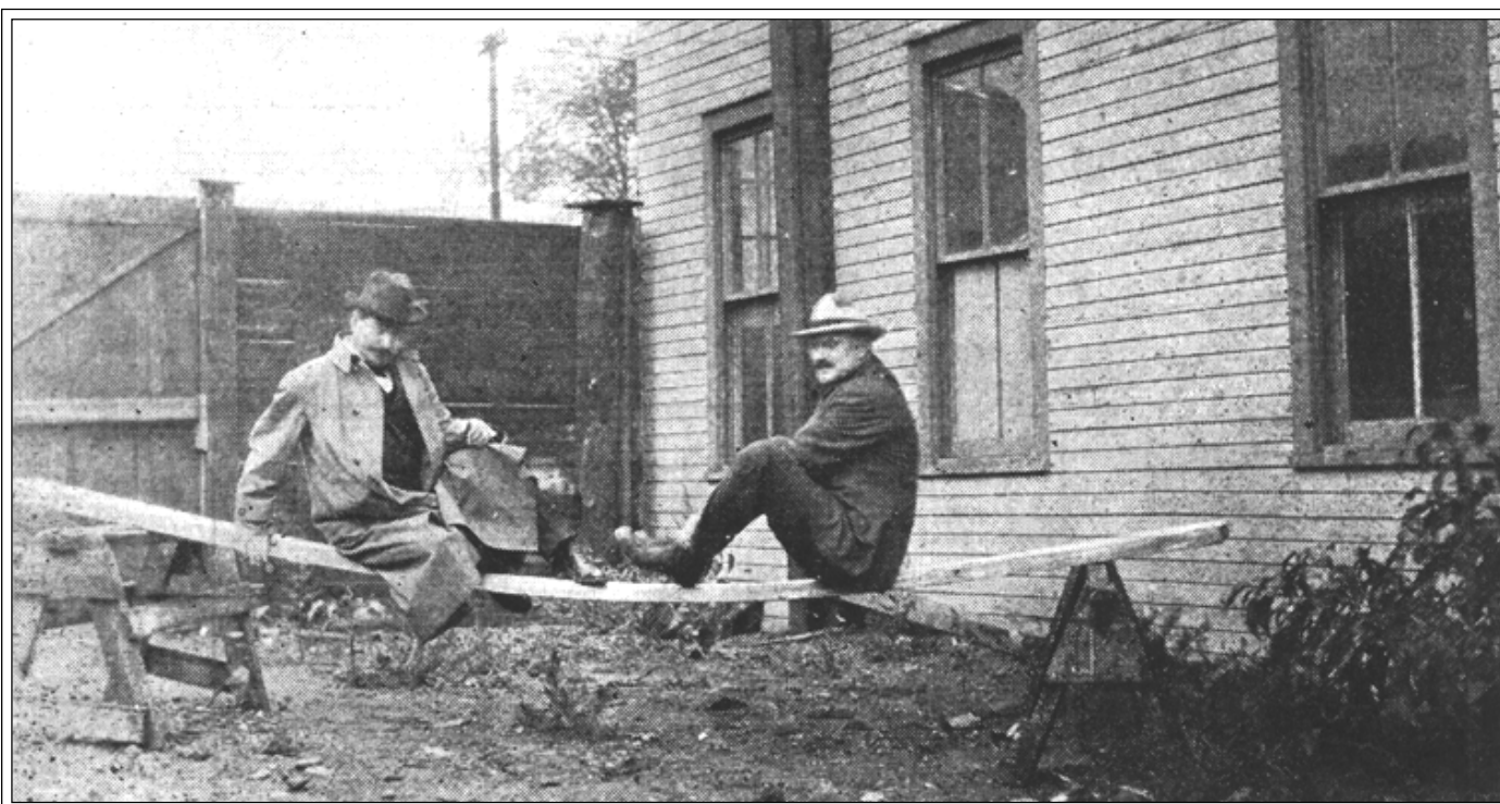
In 1917, the Journal of The American Society of Refrigerating Engineers reported tests to determine the elastic deformation of balsa wood. They were part of a study on the properties of balsa as an insulation material.
